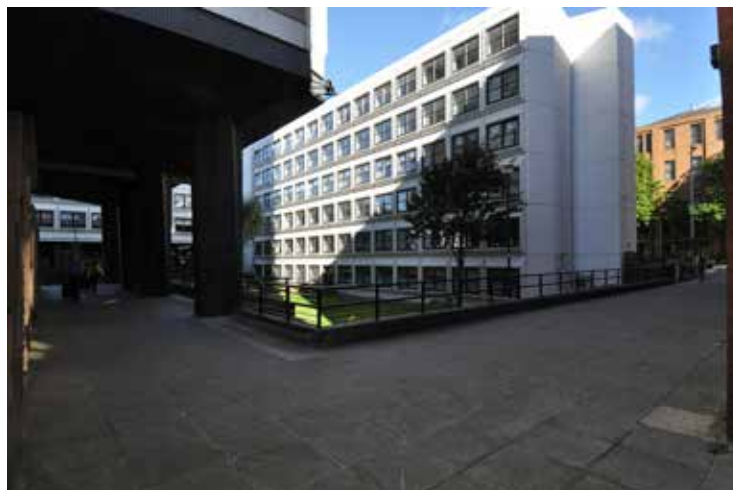
Elmbank Gardens - current situation
