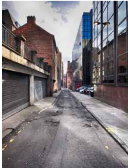
poor surfaces where yellow lining is coming off
